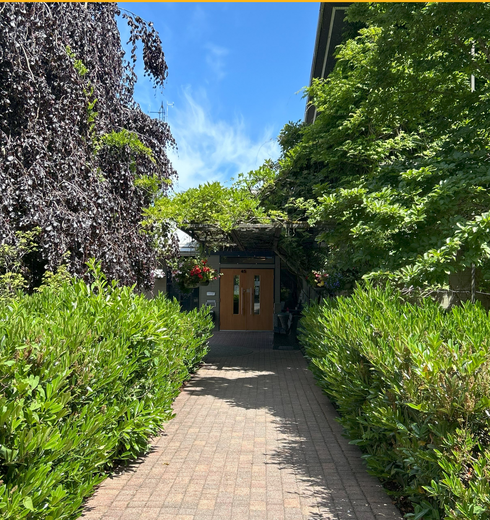
Town Hall front entrance
