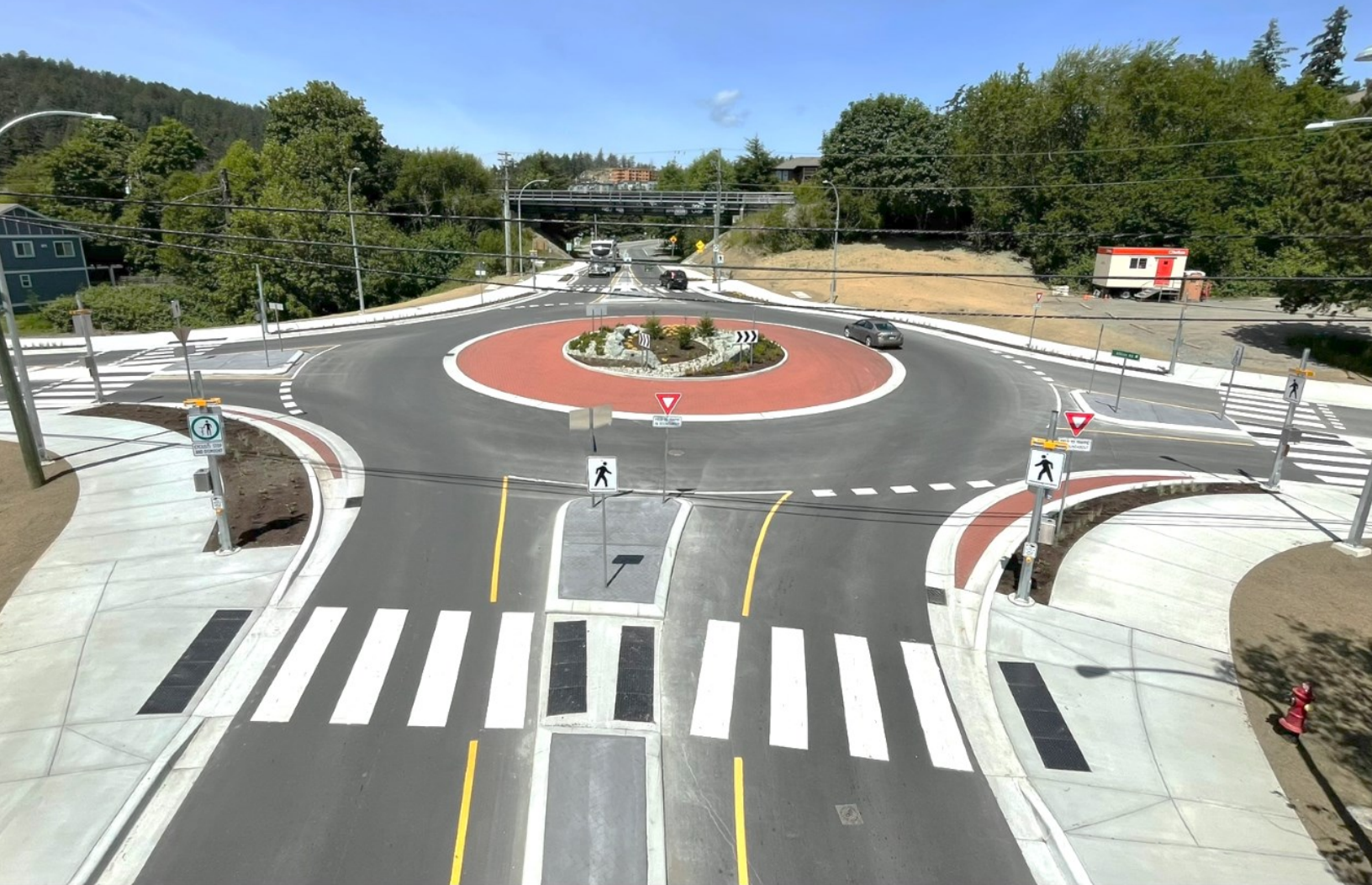
New Six Mile Road/Atkins Road roundabout
